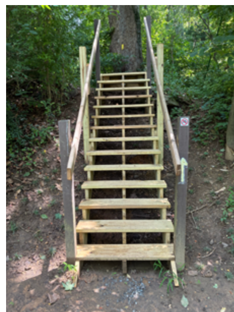
New Stairs, supported by 6x6 lumber anchored into the ground at top and bottom
