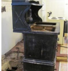
The stove as it is removed from the kitchen, showing the hole in the floor for coal ash waste
