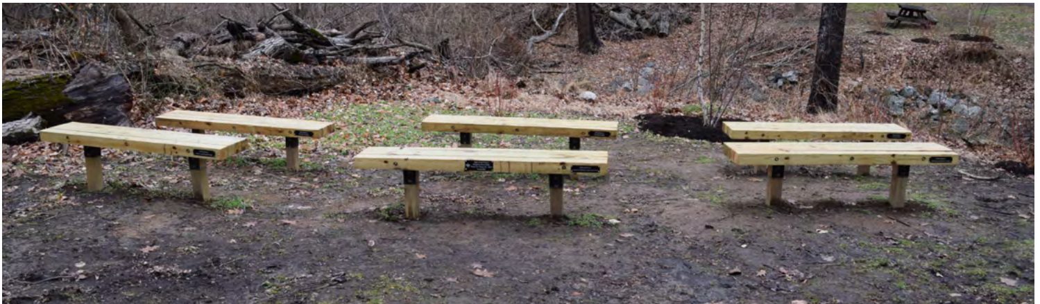
Outdoor teaching area constructed by scout Benjamin House-Kelly
