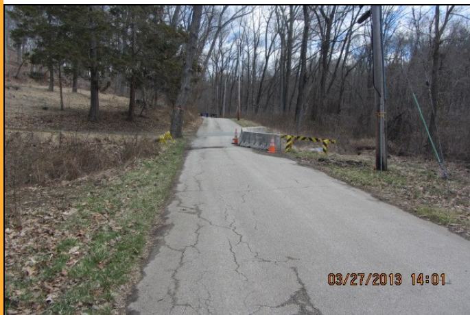
MUT Culvert Repair...Before
