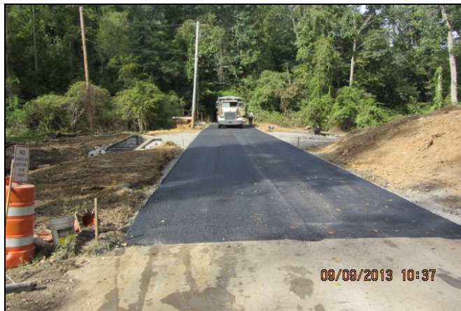
MUT Culvert Repair...After
